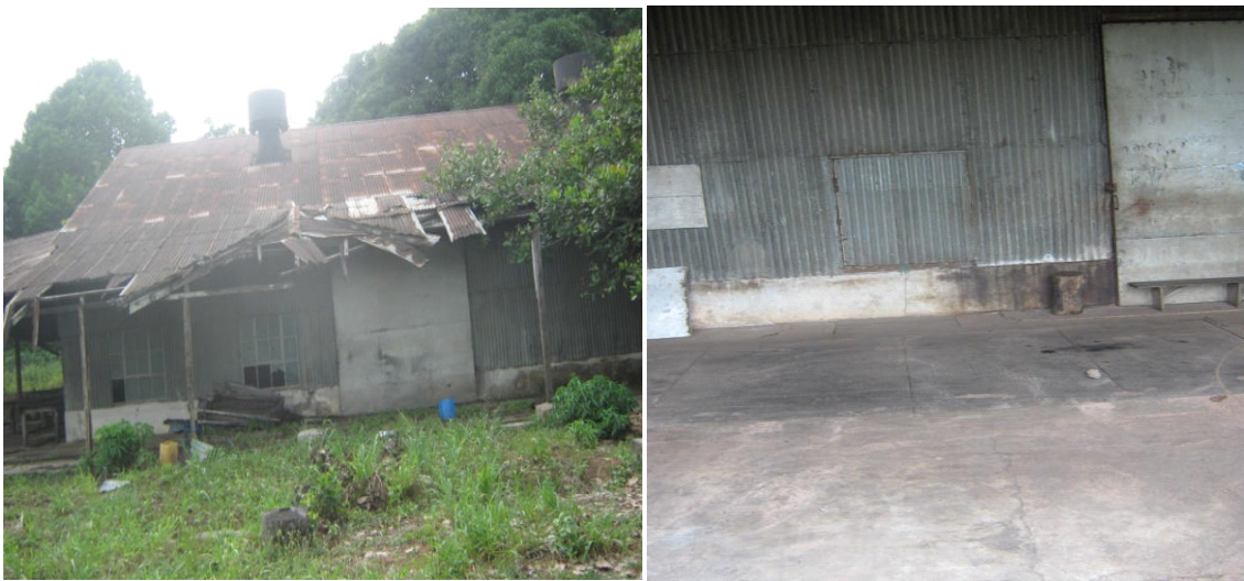
Fig 7: Side and front views of the Weigh bridge of the factory (still functional but not in use) Source: Field Survey,2012
