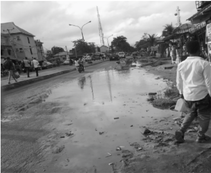
Plate 1: Showing the State of Federal Polytechnic Road
