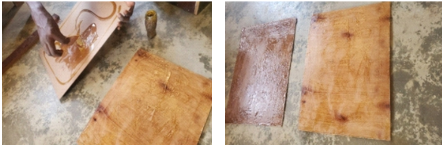
Fig. 13: Application of Evostick to the plywood
