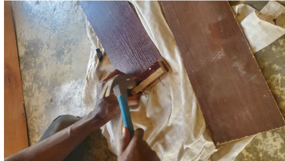
Fig. 5: Preparing the brace for the rectangular box
