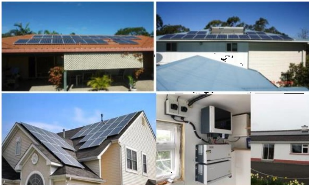
Fig. 1: Photovoltaic solar energy installations connected alongside with the batteries and inverter for residential applications (Ohwofasa, 2018).
