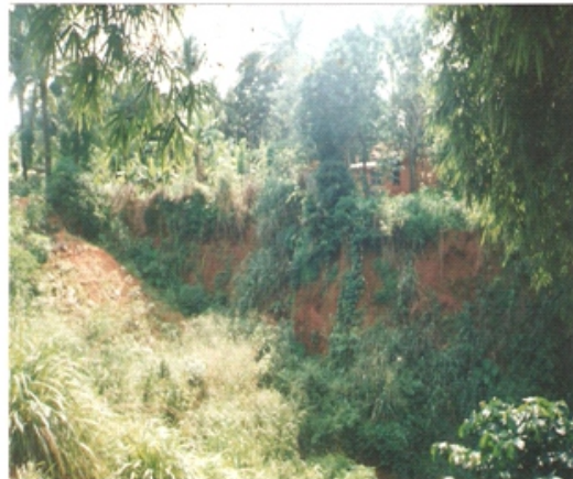
Plate 2: A House Threatened by Gully Erosion in Chikun LGA.
