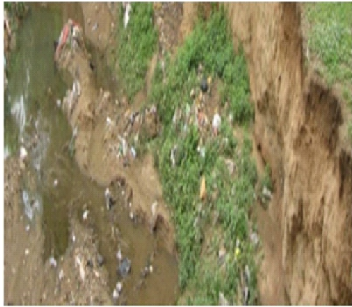
Plate 1: High Wall of Erosion Complex Source: Field Work, 2016
