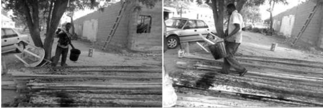
Plate 6: Minimum Preservative Chemical Treatment of Timber by Brushing during the Reconstruction of School of Environmental Studies Complex
