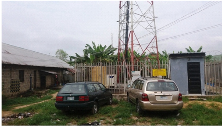
Telecommunication mast in a residential building at Efeke-Ama, Amassoma
