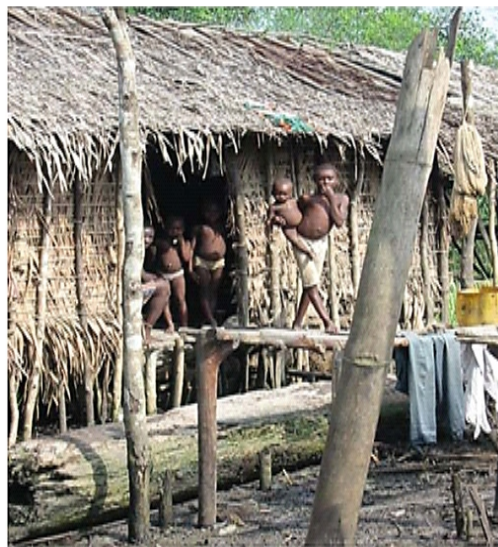
Figure 2: Burutu community in Delta State where there is complete absence of basic social amenities (infrastructure)
