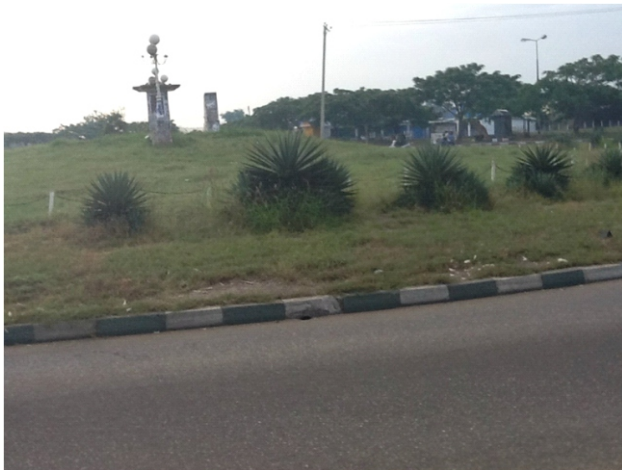
Plate 012; Unkempt roundabout. A round-a-bout is expected to be beautified to serve as tourist attraction
