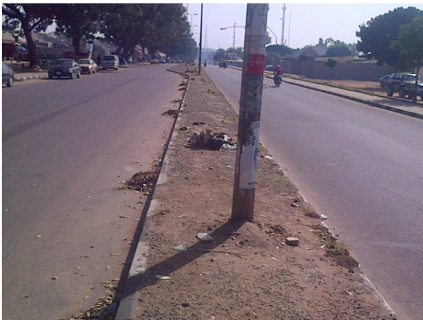
Plate 010; Untidy road divider of a major street
