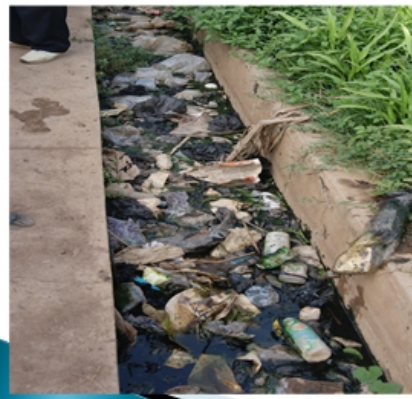
Plate 5. Drainage channel blocked by waste at Obate area of Osogbo Source: Authors Field Survey, 2019
