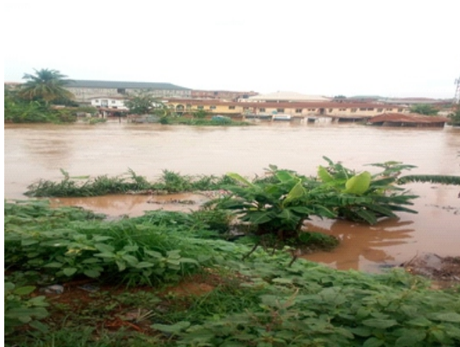
Plate 3: Buildings constructed along the flood plain in Gbodofon area of Osogbo. Source: Authors Field Survey, 2019
