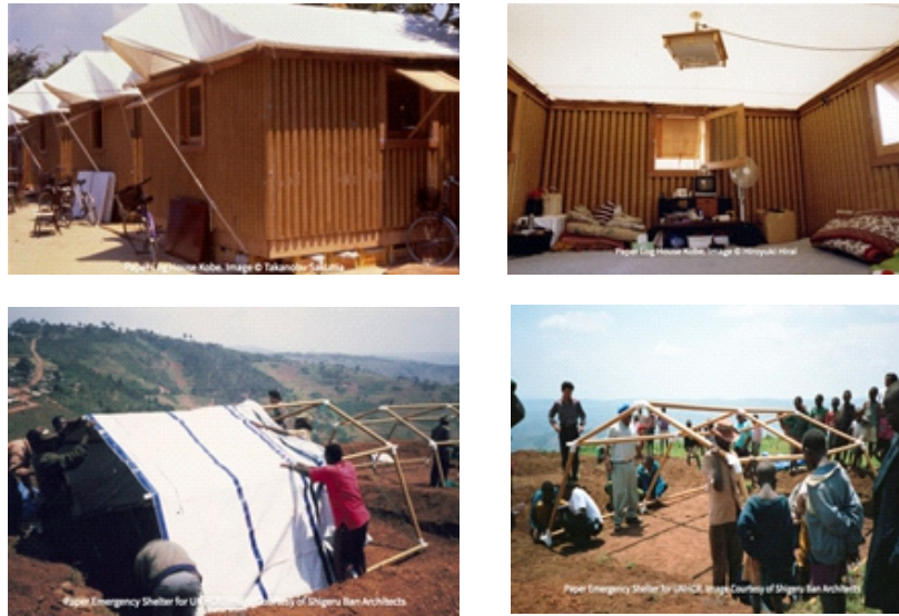
Plates 5-8 (Clockwise from top left): exterior of Shigeru Ban's recycled paper log houses in Kobe, Japan (1995); interior of paper log house; paper log framework assembly in Byumba refugee camp, Rwanda (1999); tent covering of the paper log tents
