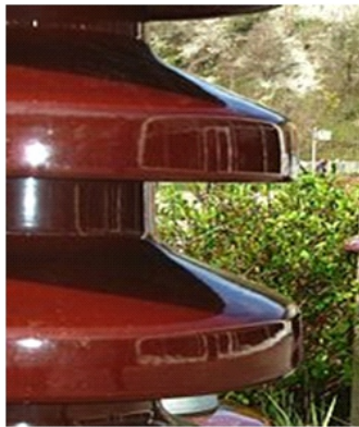
Plate 10: Porcelain High-Voltage Insulator (Wikipedia, 2016)
