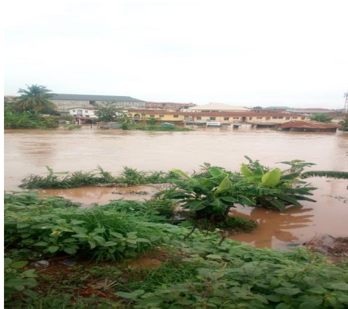
Plate 3: Buildings constructed along the flood plain in Gbodofon area of Osogbo.
