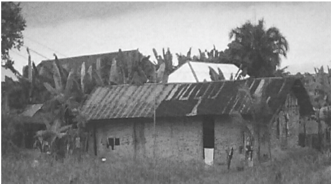
Figure 8: A family house in an Oil Producing Community in Emeyal
