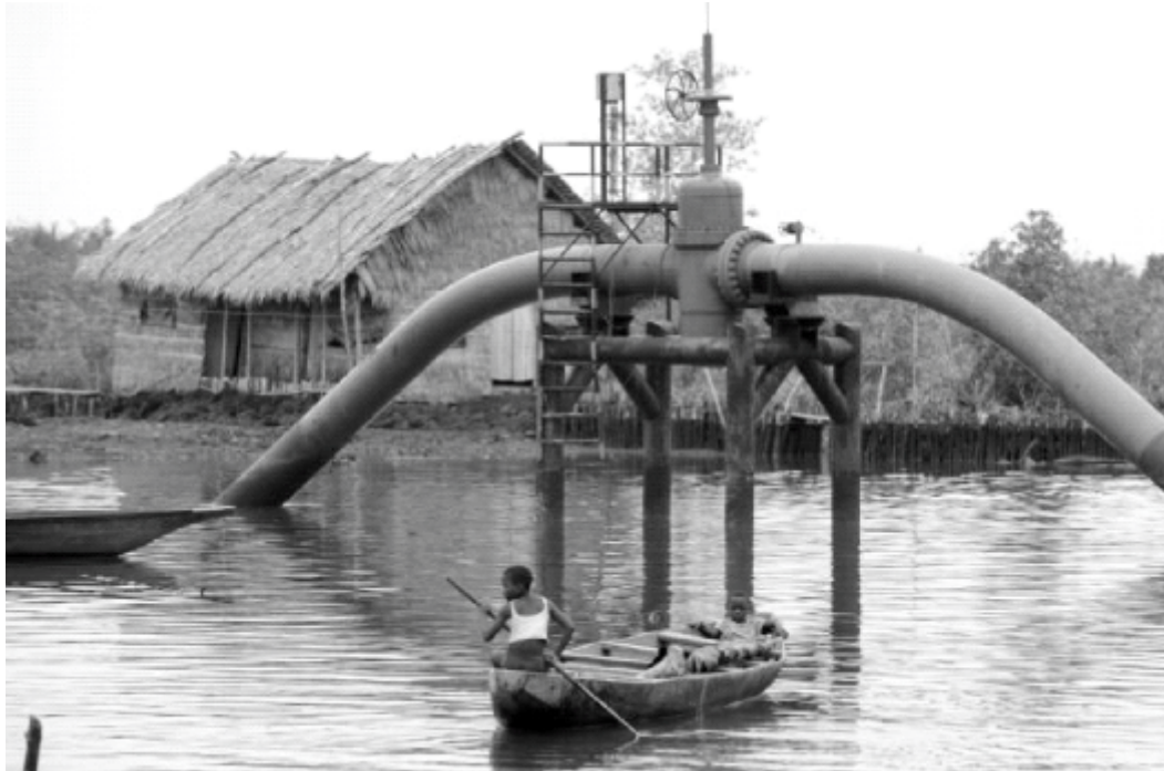
Figure 5: A Drilling Rig near a living house of a family of 6 in Emeyal
