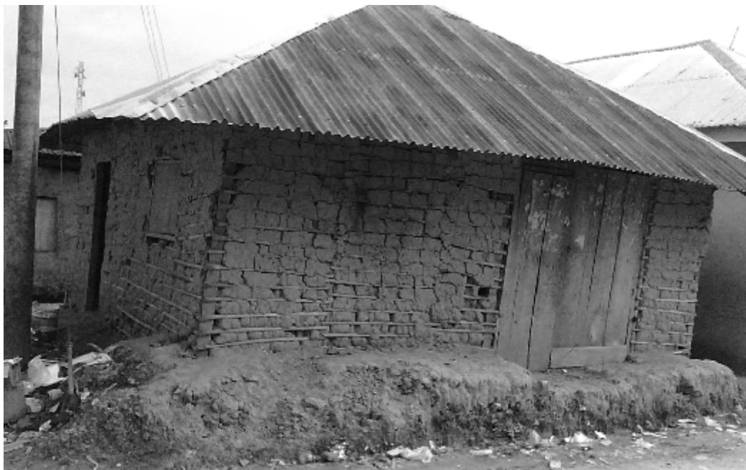
Figure 6: A family house in an Oil Producing Community in Emeyal
