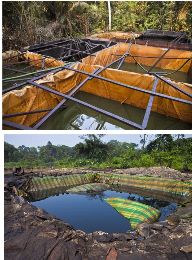
Figure 4 & 4a: Dugout Storage Facilities are laminated with Cellophane protective linings. © Timi Amah
