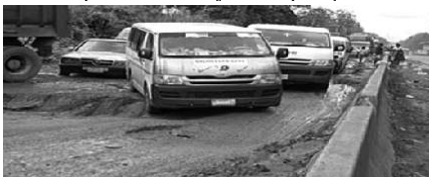
Picture 3: Collapsed and treacherous Lagos- Benin Expressway
