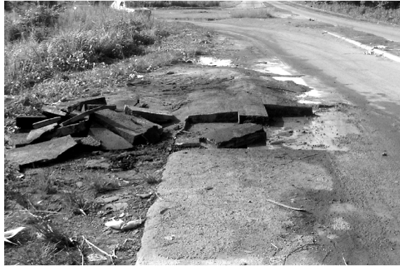
Plate 1: Cut hole around the rail line in Inisha, Osun State
