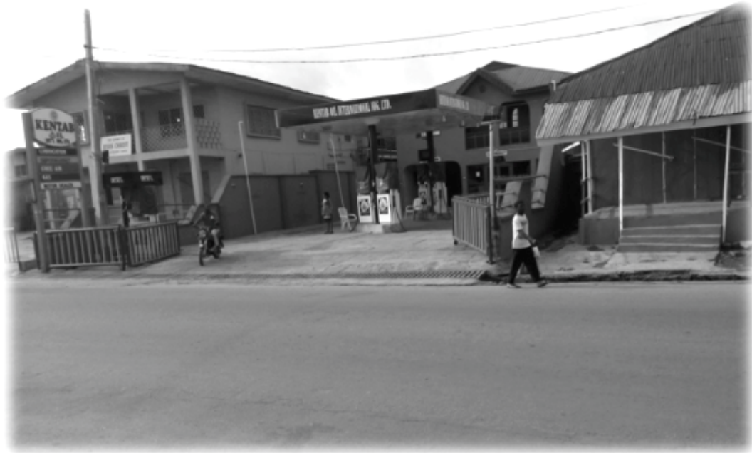
Plate 2: Violation of landmass and setback regulations
