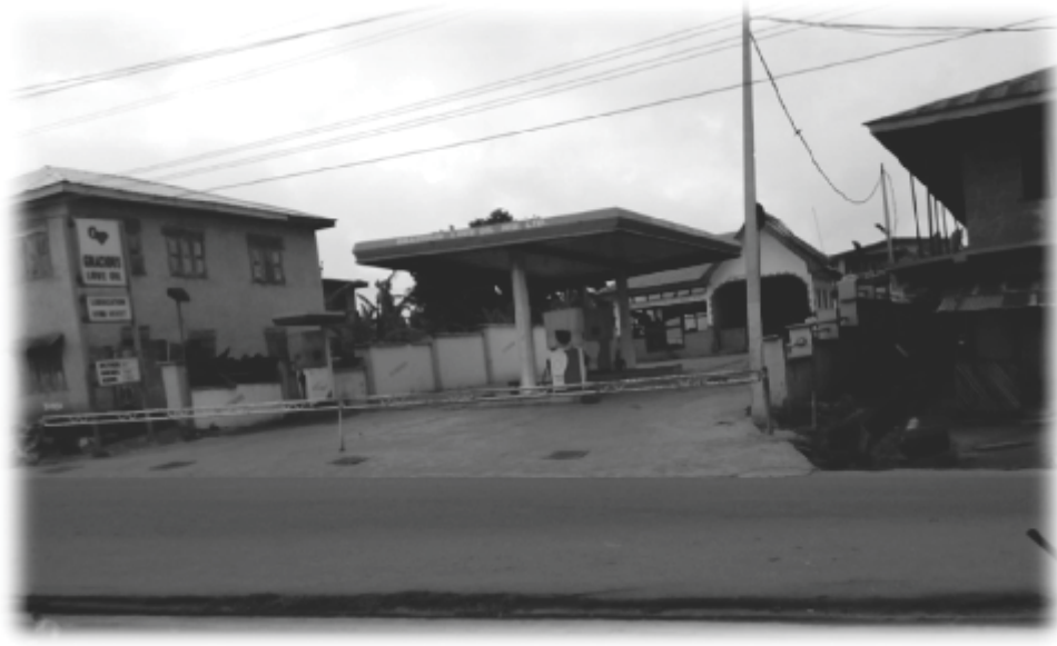
Plate 1: Violation of setback regulation to residential building
