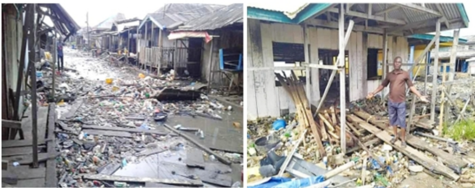
Fig 5: Destruction of buildings in the Community
