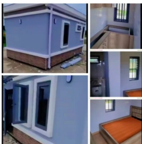
Figure 9: Exterior and interior images of 1-bedroom prototype prefab house, Abuja, Nigeria.
