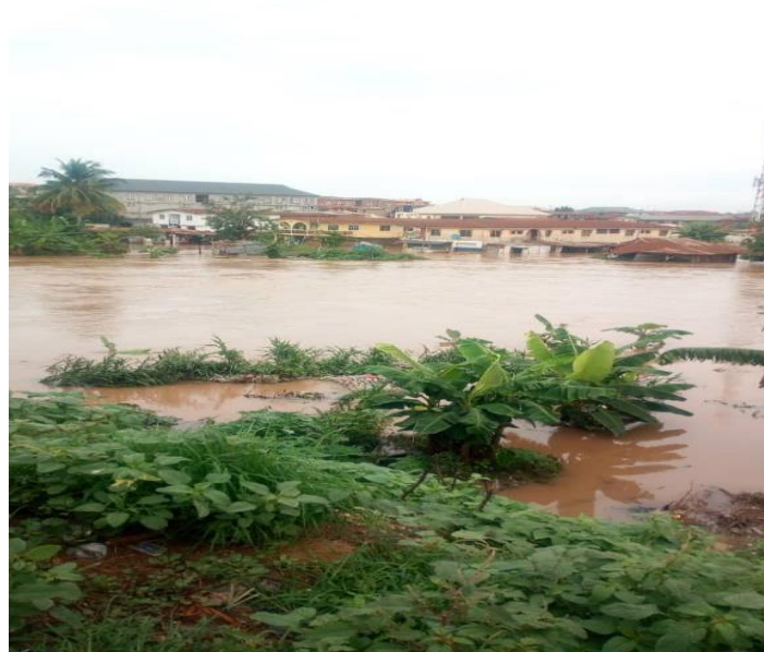
Plate 3: Buildings constructed along the flood plain in Gbodofon area of Osogbo. Source: Authors Field Survey, 2019
