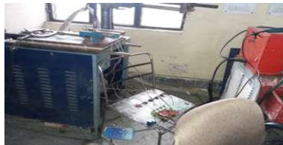
Fig 3: The complete welding set up
